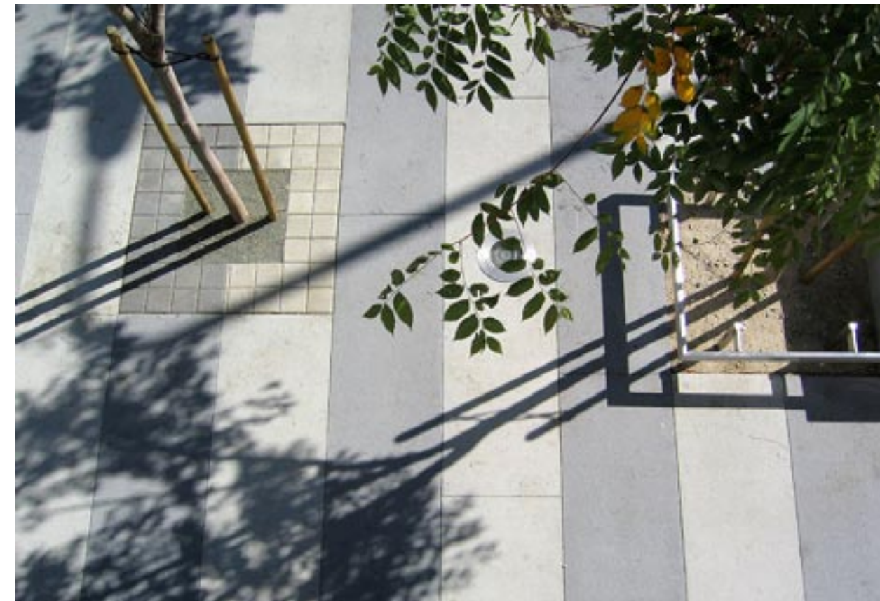
alternating bands of integrally colored concrete and D.G. treewells along Grand Avenue
