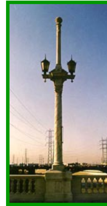
Restoration of the historic fixtures for the First St. Bridge
