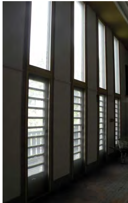
#11 – Window Columns at North Elevation
