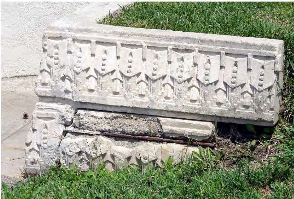
#5 – Smaller Retaining Wall at Entry
