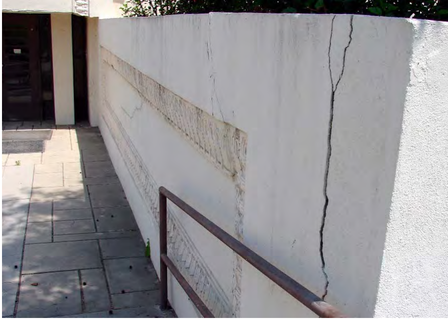
#4 – North Retaining Wall at Entry
