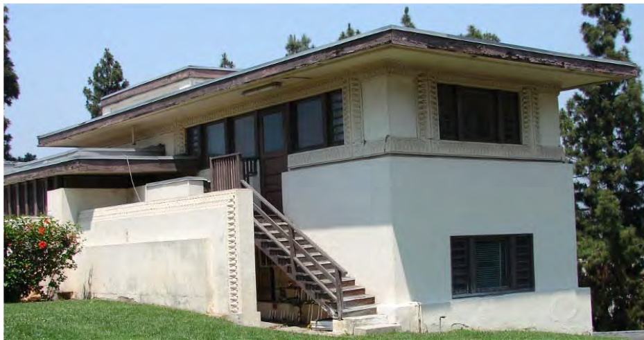
#1 – Residence A Building – South and West Elevations
