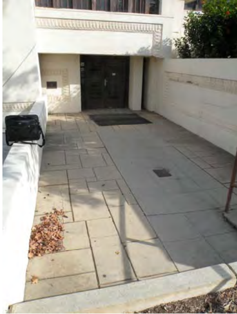
#2 – Entry Walkway and Retaining Walls
