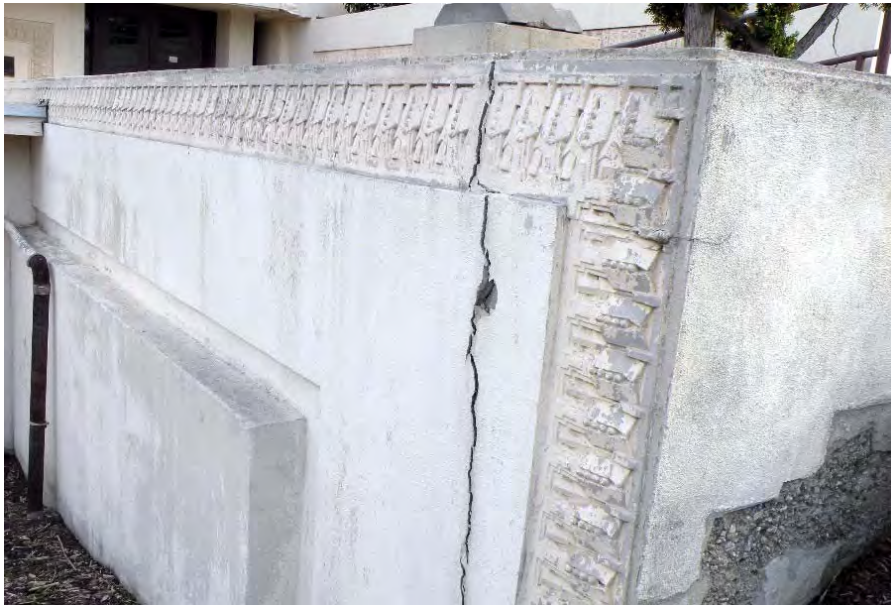
#3 – South Retaining Wall at Entry
