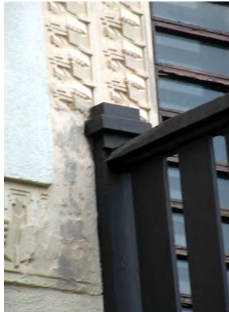
#9 – Attachment Location of Original Balcony
