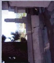
Existing tree caused patio structural damage.
