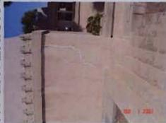
Extensive structural cracks indicated problems at the foundation level.
