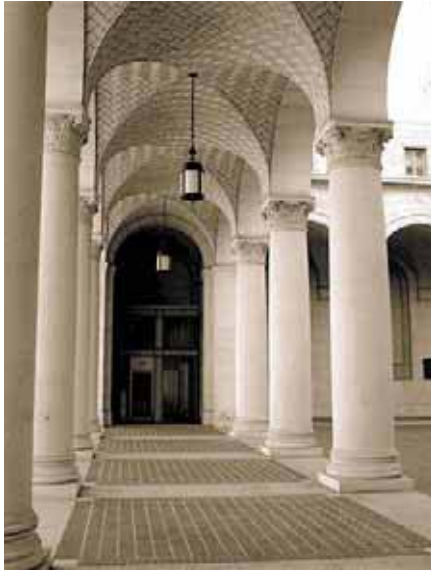
City Hall (Los Angeles) - Arcade along northern edge of west courtyard and portico
