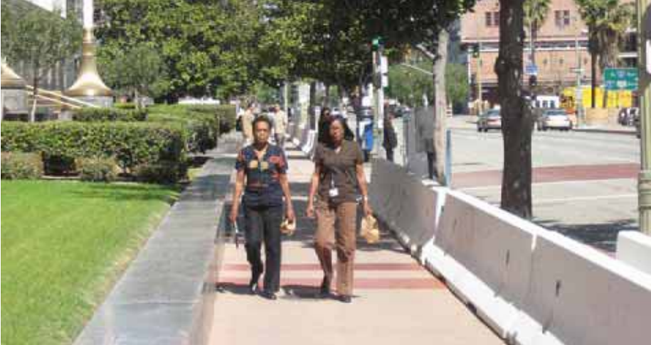
Main Street at United States Courthouse Concrete barriers, stone retaining wall, lawn
