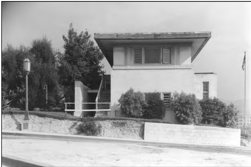
Figure 22: 1965 photo of south elevation, view north. (Photo credit: Marvin Rand, Historic American Buildings Survey)
