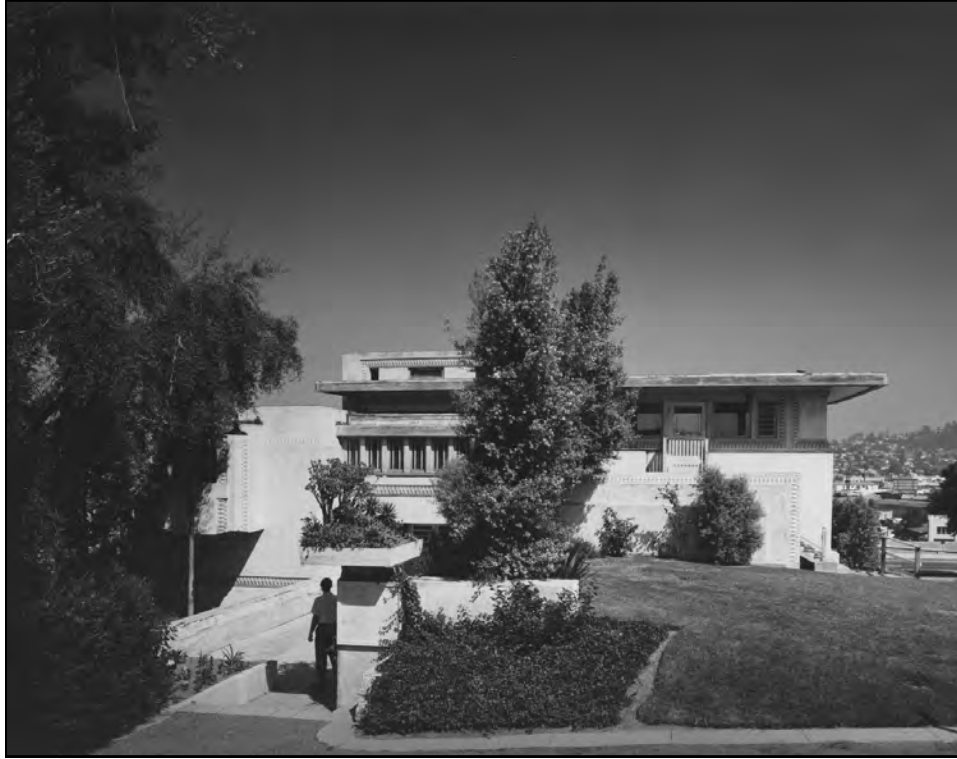
Figure 17: 1965 photo of west elevation, view northeast. (Photo credit: Marvin Rand, Historic American Buildings Survey)
