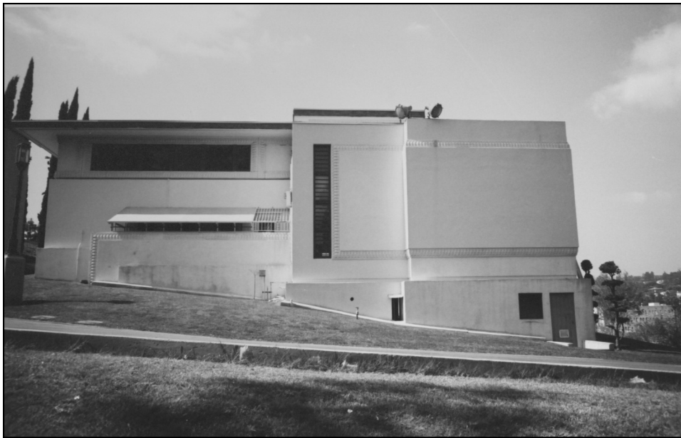
Figure 28: East elevation, view west. Photo taken ca. 2005. (Photo credit: Thomas Koester for the Aline Barnsdall Complex National Historic Landmark Nomination)
