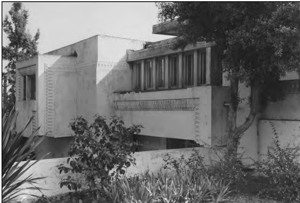
Figure 18: Detail of kitchen windows above entrance, photo taken in 1965. (Photo credit: Marvin Rand, Historic American Buildings Survey)
