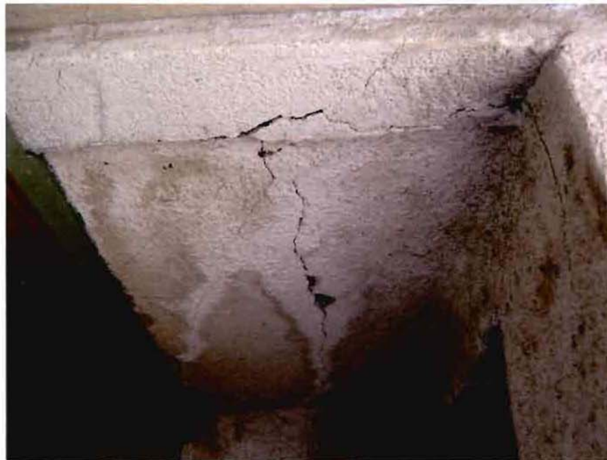
PHOTO 24 - Concrete Column & Ceiling at Line E/6
