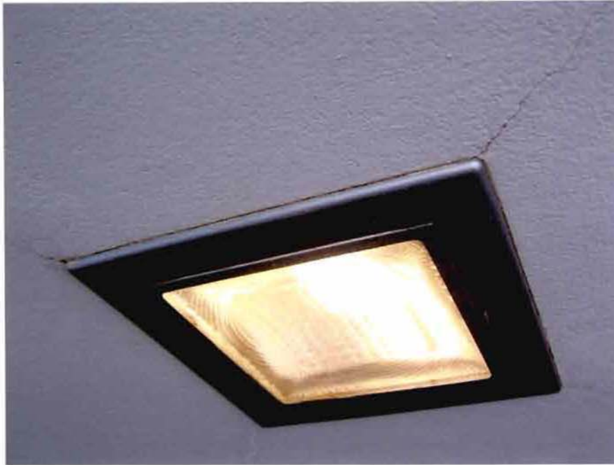
PHOTO 21 - Porch Ceiling Light at Line D.4/6.3
