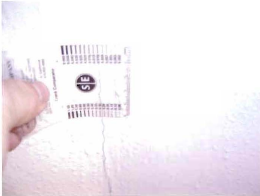
PHOTO 1 - Dining Room Interior Ceiling at Line F.5/5 to 6
