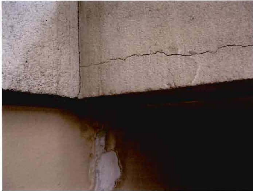
PHOTO 13 - Gallery Room Exterior Wall at Line C/6
