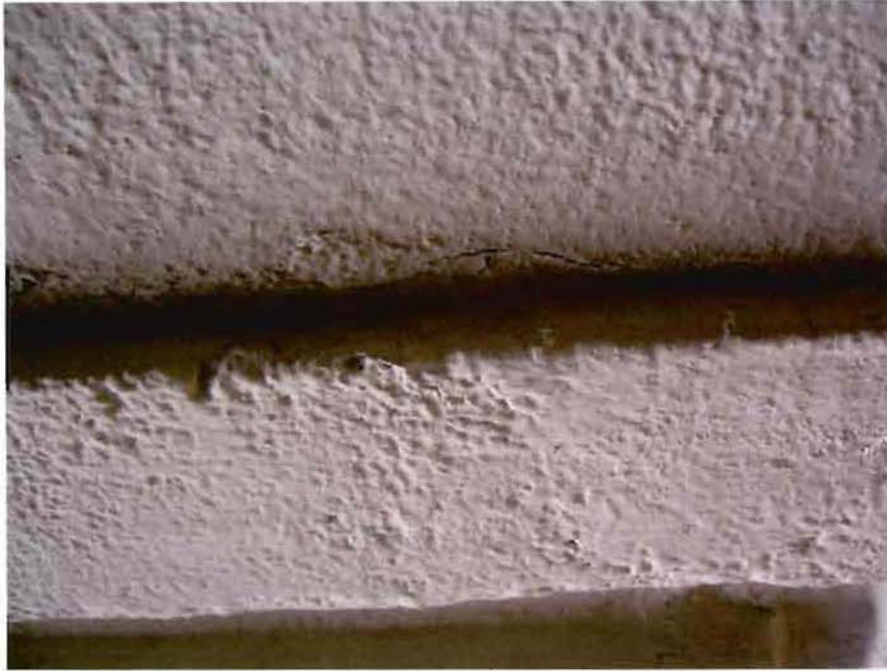
PHOTO 19 - Porch Ceiling at Line E/7
