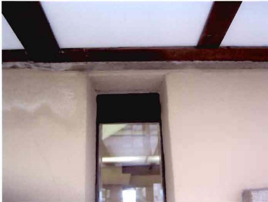
PHOTO 12 - Gallery Room Exterior Wall at Line C/5.2
