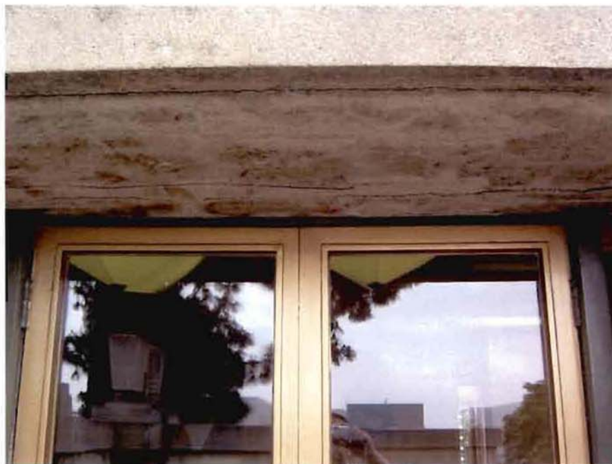
PHOTO 16 - Gallery Exterior Ceiling Above Window at Line B/5.5
