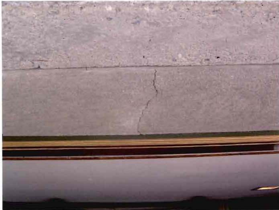
PHOTO 25 - Ceiling Above Door Entrance at Line 6/D.5
