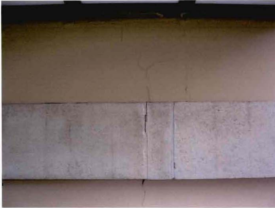
PHOTO 15 - Gallery Room Exterior Wall West of Door at Line C/4
