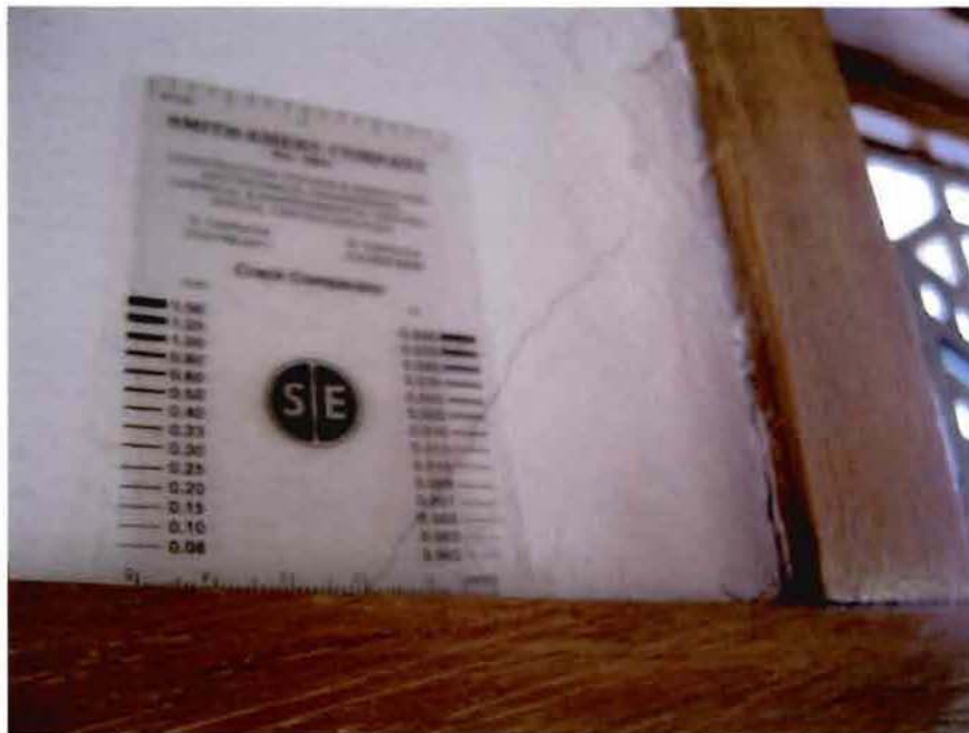
PHOTO 6 - Dining Room Interior Walls at Line H/6
