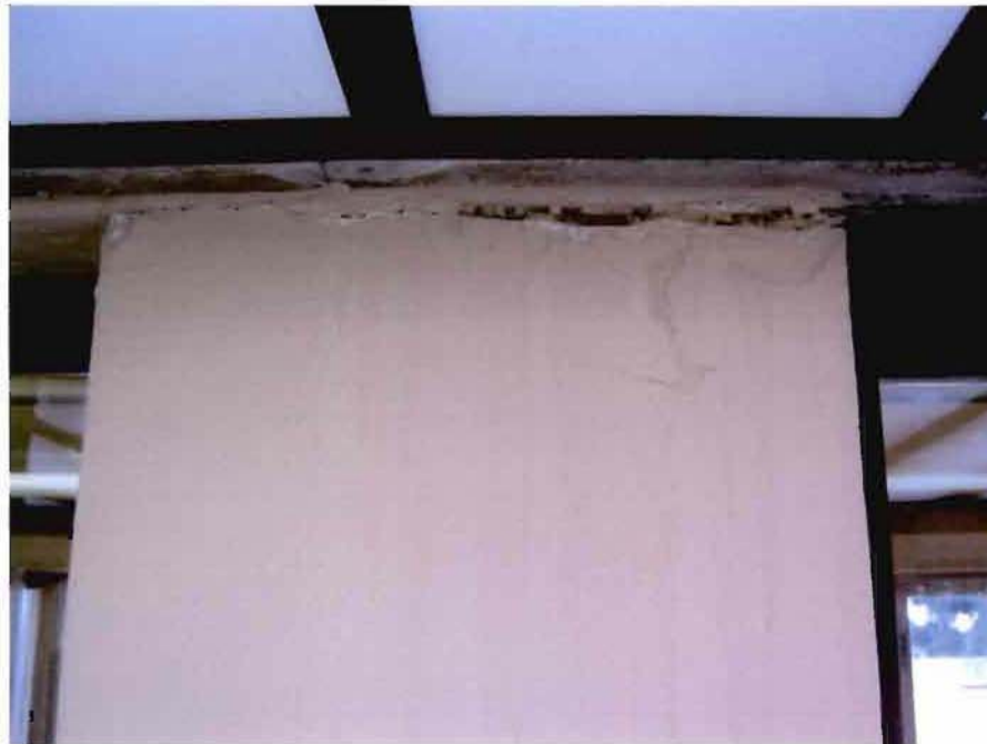
PHOTO 14 - Gallery Room Exterior Wall at Line C/4.7
