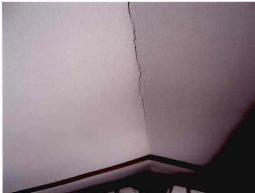
PHOTO 2 - Dining Room Interior Ceiling at Line F.5/5 to 6
