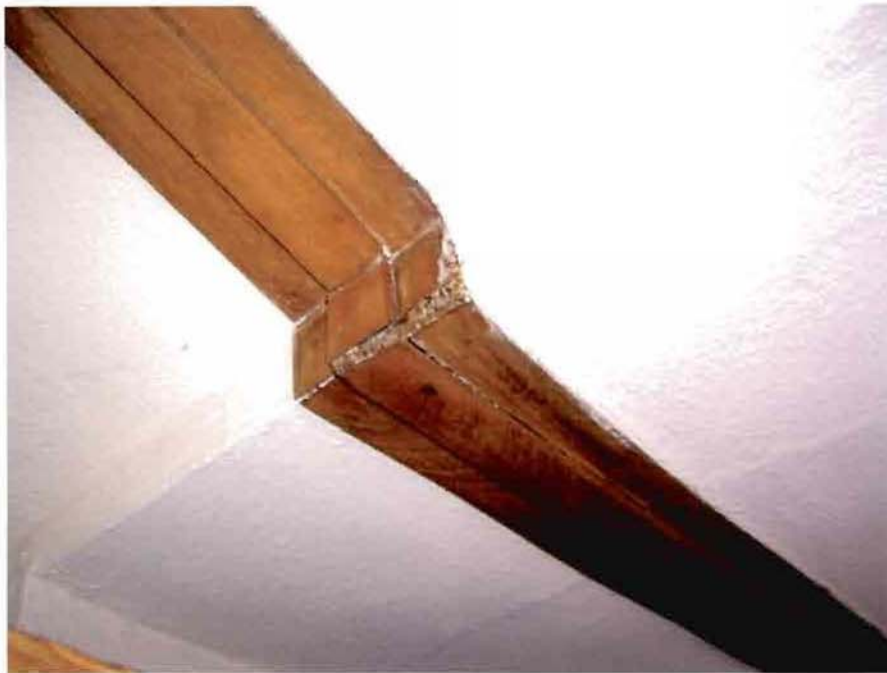
PHOTO 3 - Dining Room Interior Ceiling at line G/6.2
