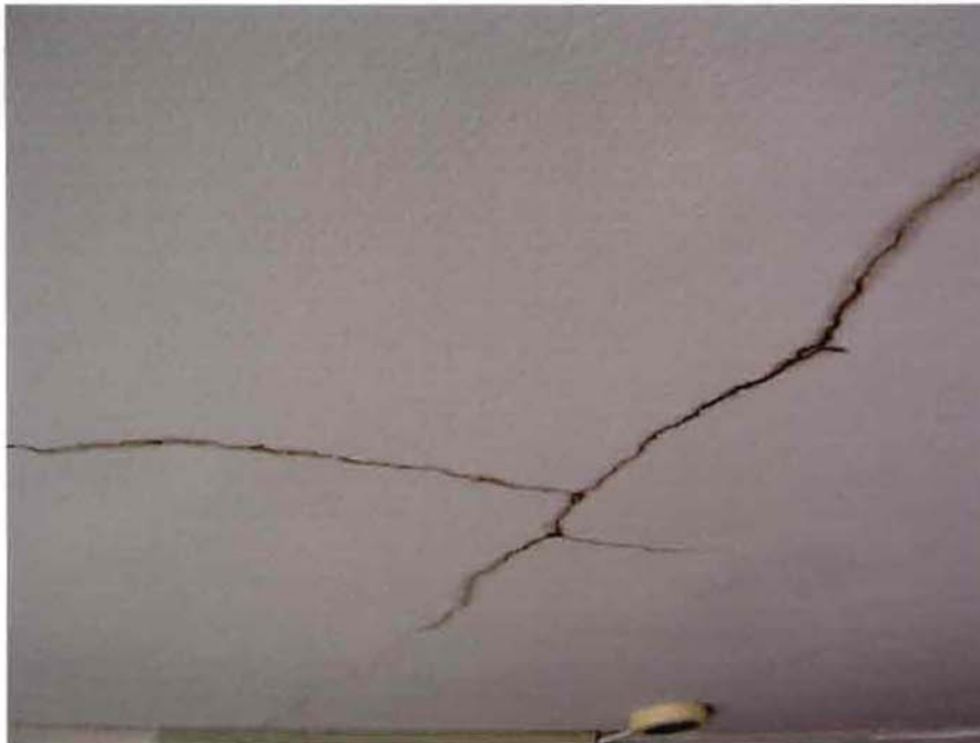
PHOTO 20 - Porch Ceiling at Line D.2/6.2
