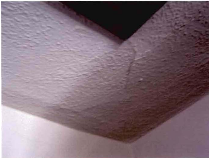
PHOTO 4 - Dining Room Interior Ceiling Test at Line H/5
