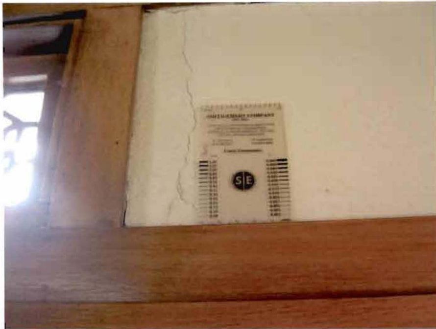
PHOTO 7 - Dining Room Interior Walls at Line 6.2/G.5
