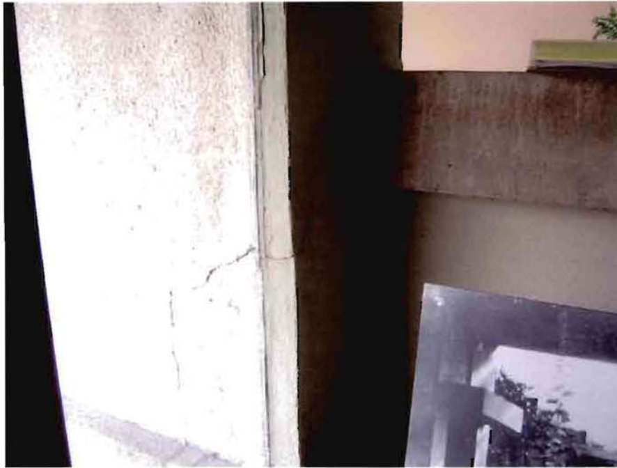
PHOTO 23 - Concrete Column at Line D/6
