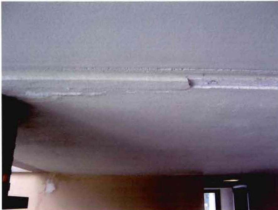
PHOTO 22 - South Entrance Ceiling at Line D/6.5 to 7
