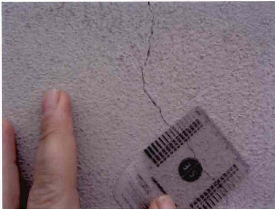
PHOTO 9 - Dining Room Roof at Exterior Parapet Wall at Line F/4 to 6
