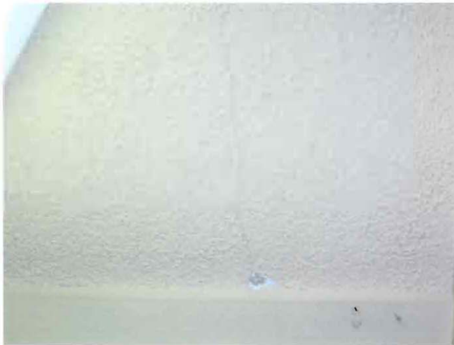
PHOTO 10 - Gallery Room Interior Ceiling at Line B to C/ 4 to 6
