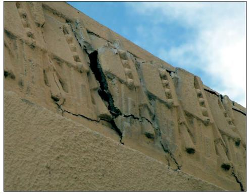
**Figure 18:** Typical decorative cast stone damage. (Photo credit: CK Arts, 2008)
