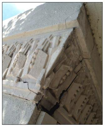
**Figure 17:** Damaged decorative cast stone at balcony. (Photo credit: CK Arts, 2008)
